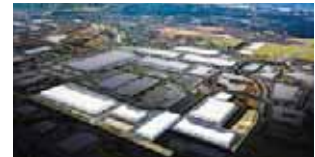
PACIFIC GATEWAY INDUSTRIAL PARK Kent, WA 823,600 SF
